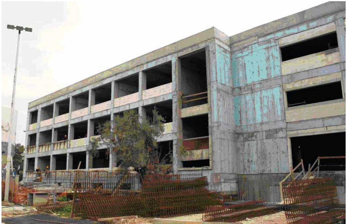
During Construction of Building A'
