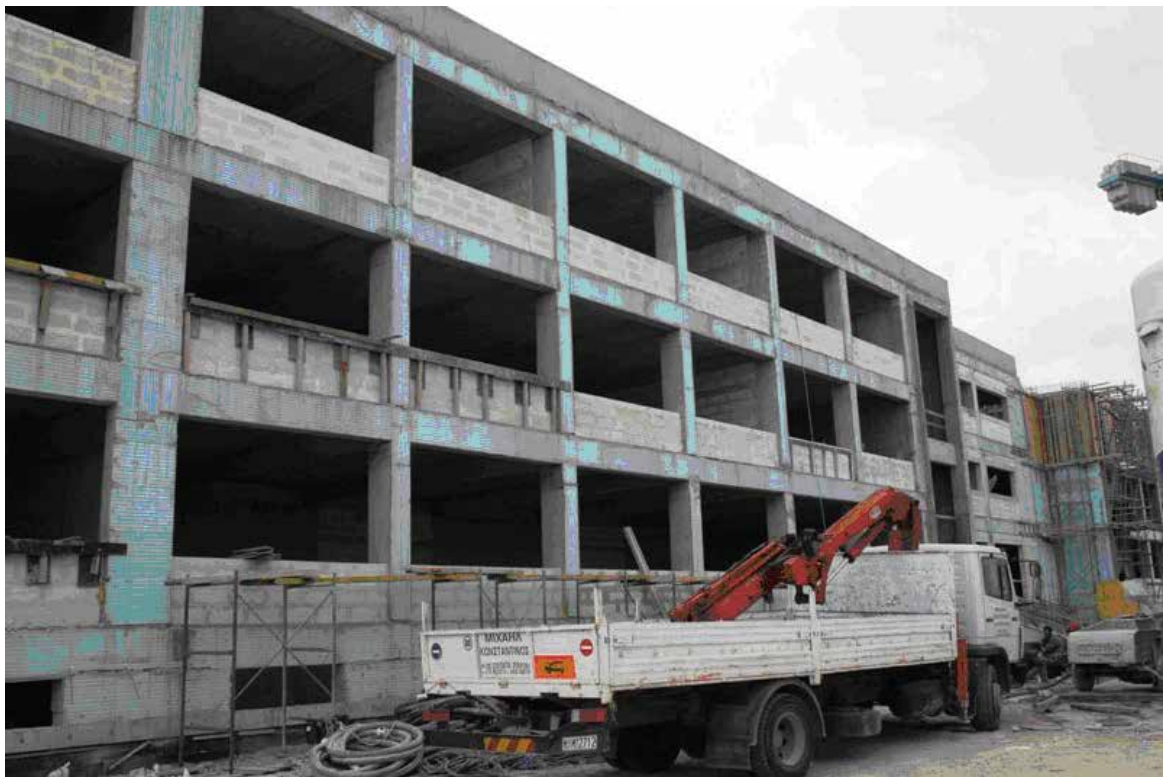
During Construction of Building B'
