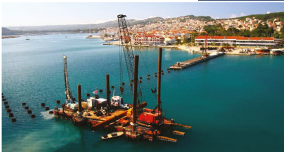
Argostoli cruise vessels berth - Construction phase
